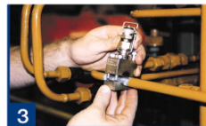
clamp SC onto pipe
