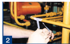
remove paint and clean pipe
