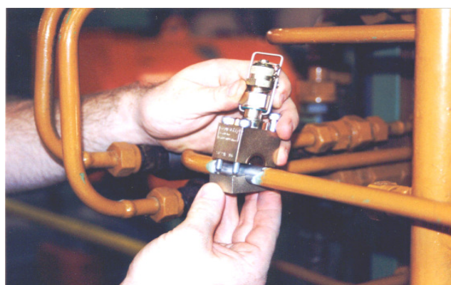
Installation on non-pressurized pipe serv-Clip® 2
